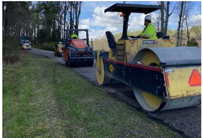
Rolling of the chip seal
