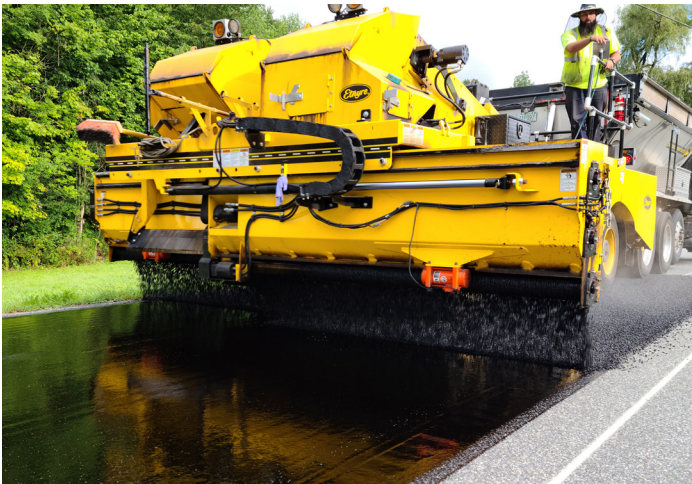
Application of the 7/16" cover aggregate
