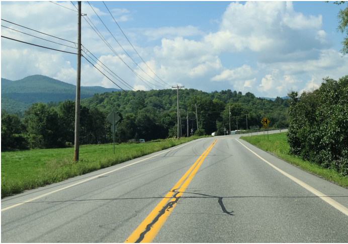
Pre-existing condition of the roadway
