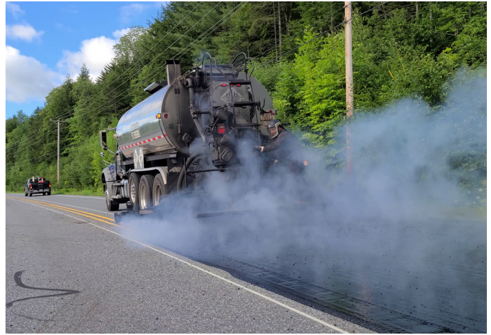
Application of the asphalt rubber binder
