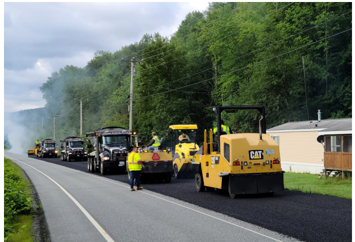
Rollers following directly behind the chip seal application
