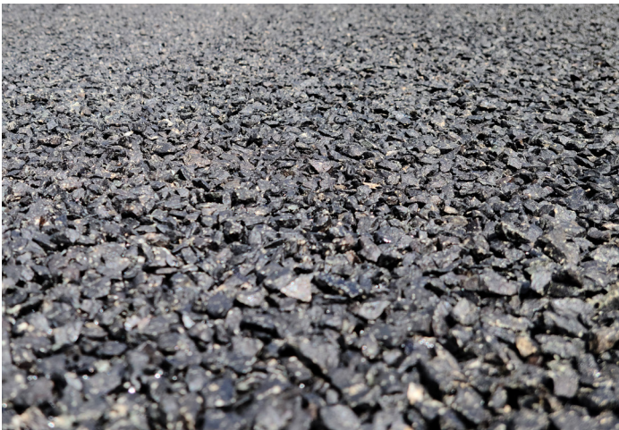
Close up of the chip seal surface after sweeping
