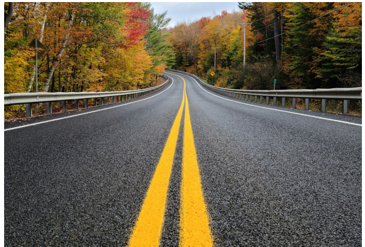
Completed and striped chip seal surface
