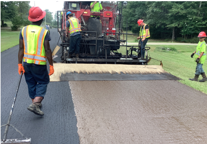
Application of the second half of the roadway
