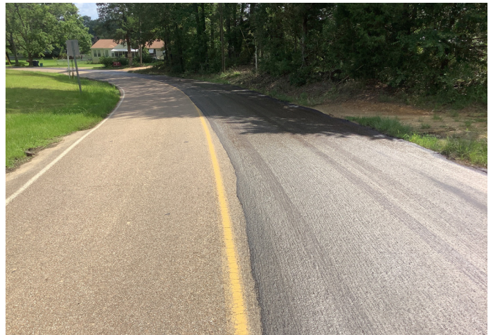
Cured view of the first half of the roadway
