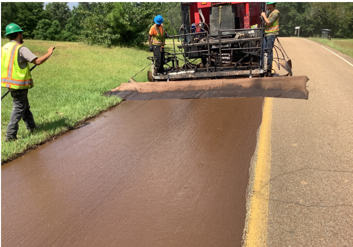
Application of the first half of the roadway
