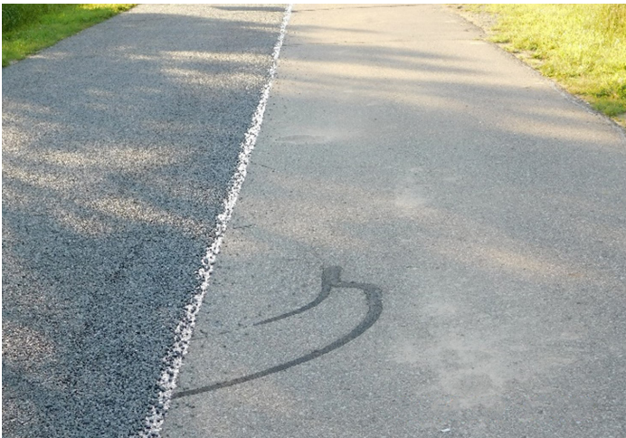
Chip completed on one half of the roadway
