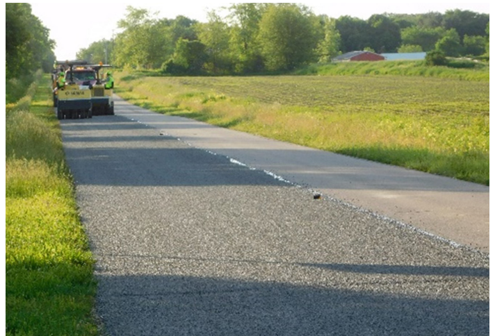
Rolling of chip sealed surface
