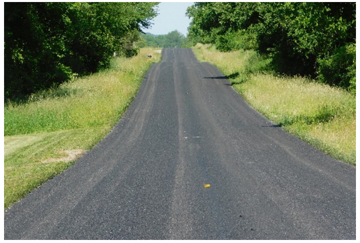
Completed surface following fog seal
