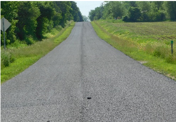
Completed chip seal prior to fog seal
