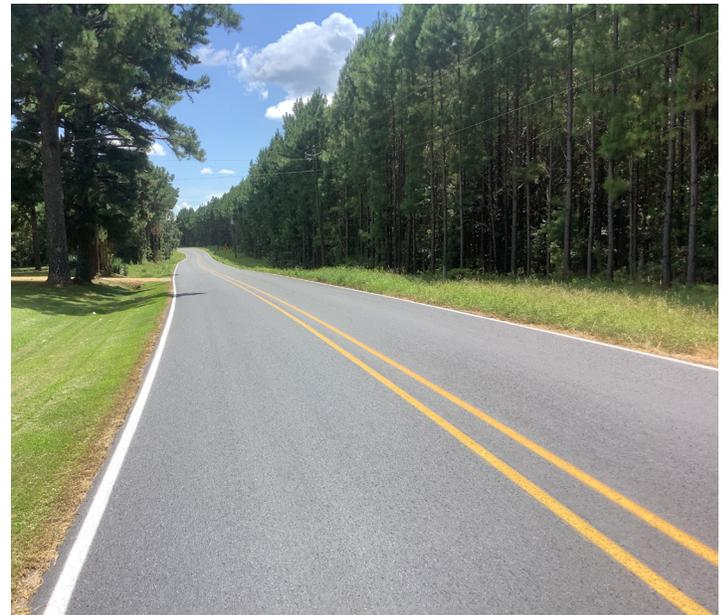
The project scope included surface preparation, calibration of the materials, and the placement of Type II micro surfacing.
