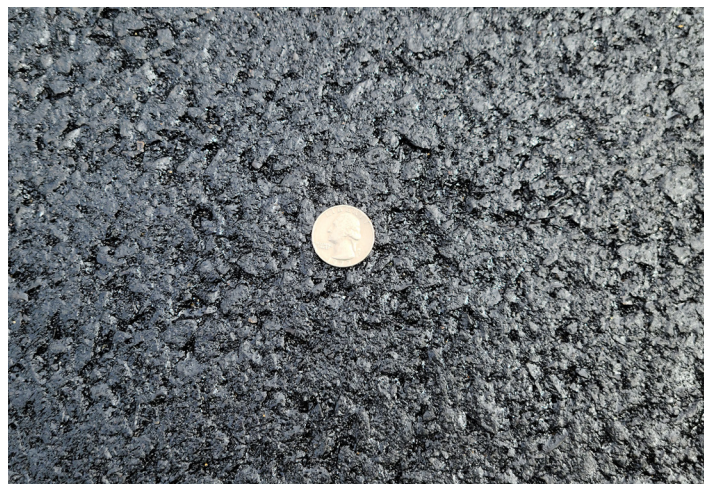
Close-up view of cured Fog Seal surface after one day
