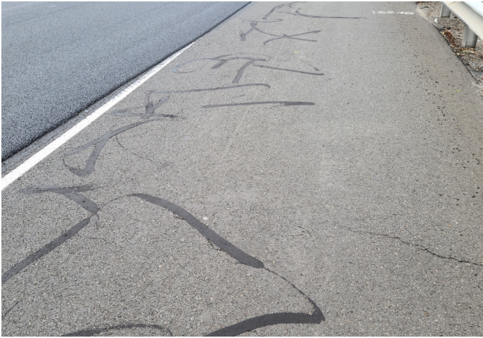
Pre-existing shoulder surface condition
