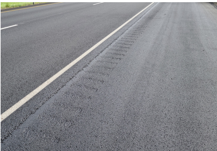
Cured Fog Seal one day after application
