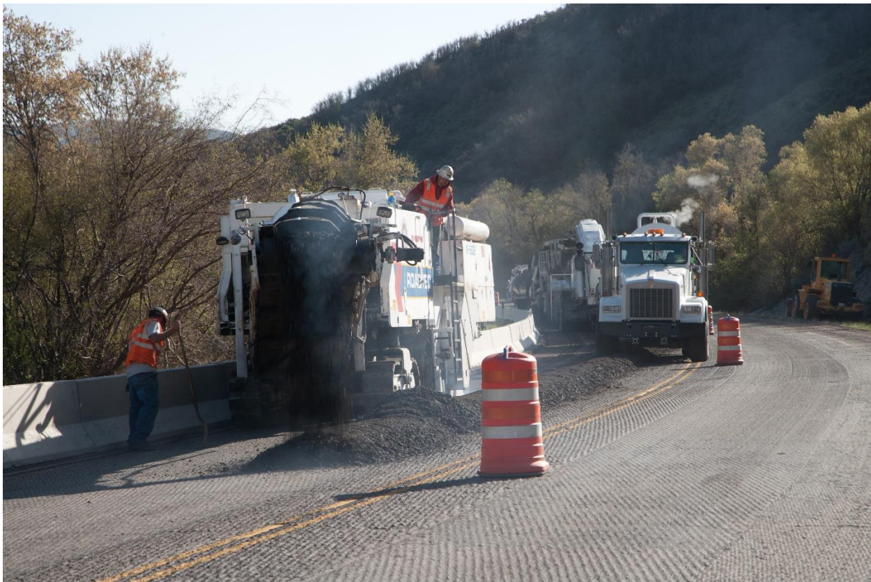
Figure 9 Recycling the shoulder plus full lane width by using a second milling machine. (courtesy ARRA)
