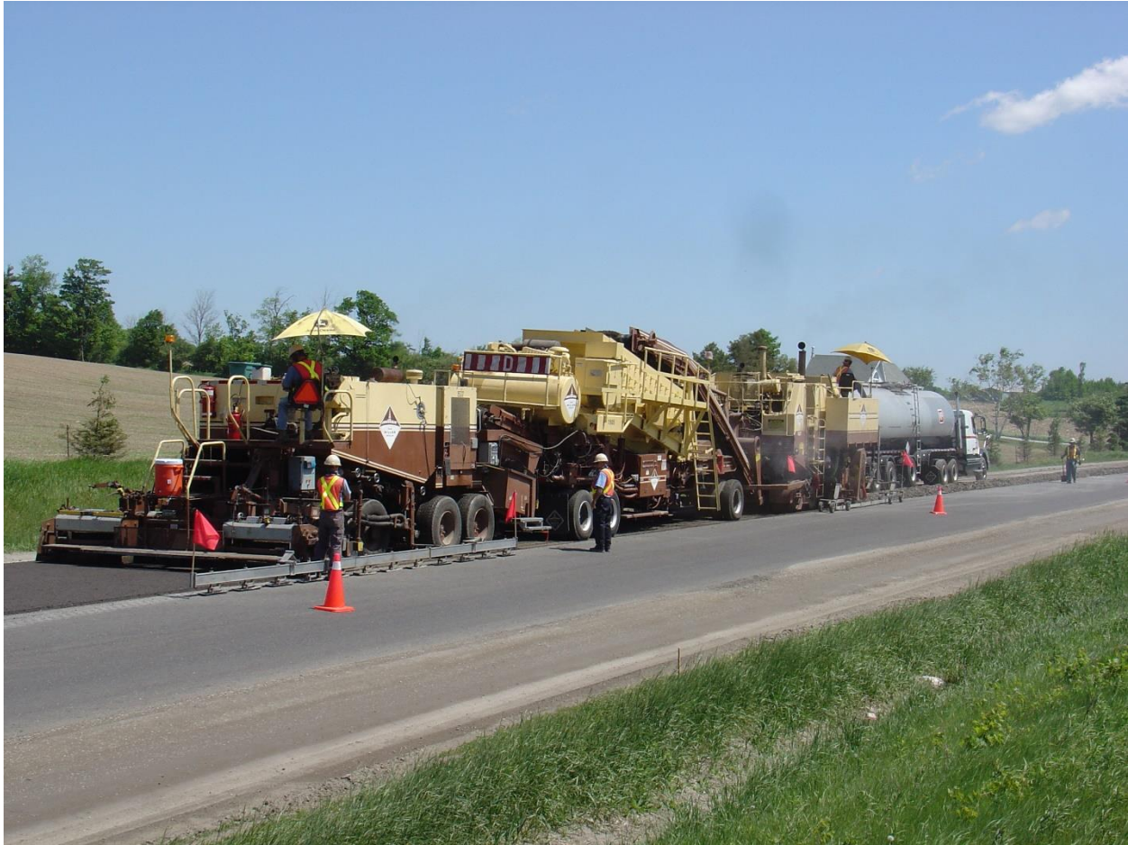
Figure 16 Multi-unit train (courtesy ARRA)
