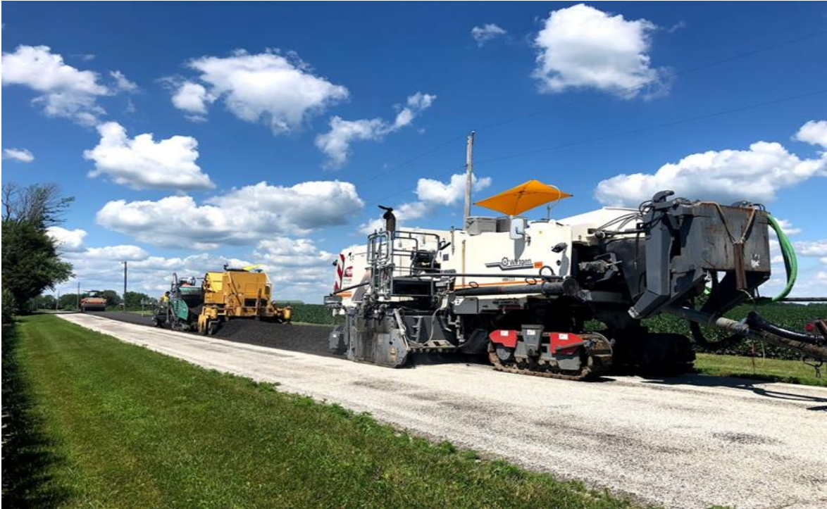
Figure 23 CCPR Mix Being Delivered to Paver via Windrow (Courtesy HRG)
