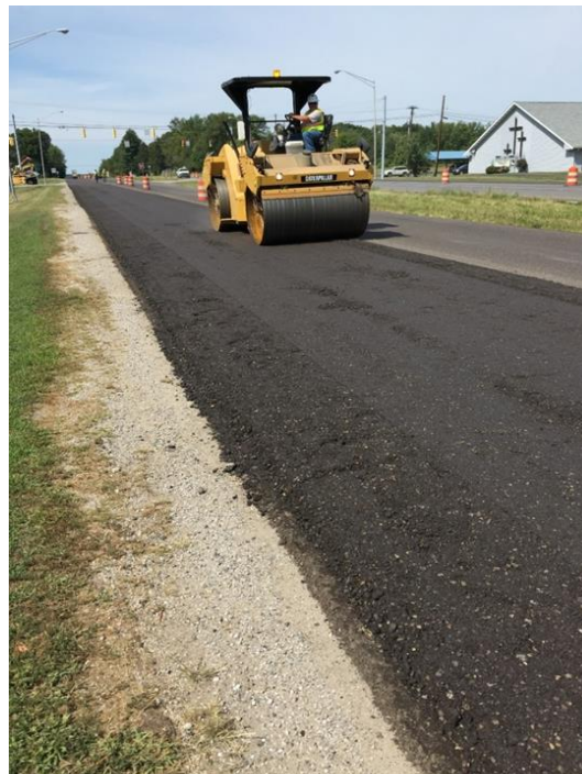
Figure 21 Minimum 10 ton Vibratory Roller (Courtesy HRG)
