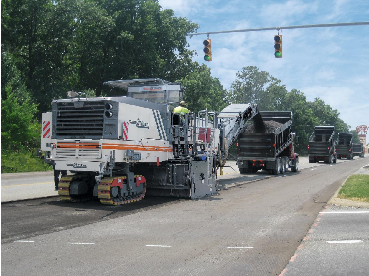
Figure 10 Milling machine depositing RAP into haul trucks. (courtesy ARRA)
