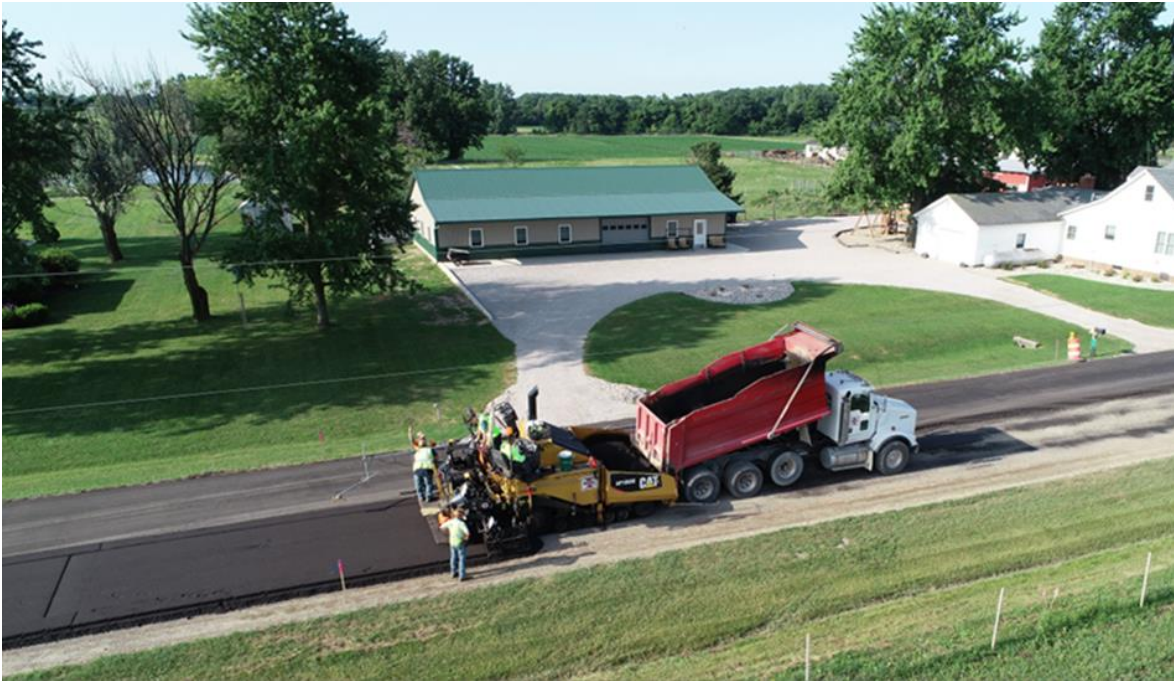
Figure 24 CCPR Mix Being Directly Delivered to Paver (Courtesy HRG)
