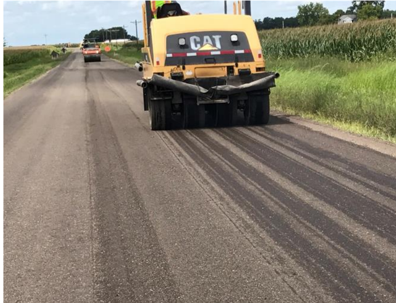
Figure 20 Minimum 22 ton Pneumatic Tire Roller (Courtesy HRG)
