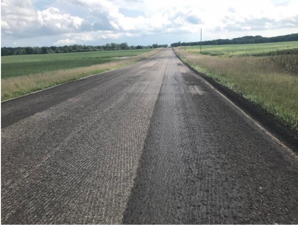
Figure 26 CCPR After Scarification Milling (Courtesy HRG)
