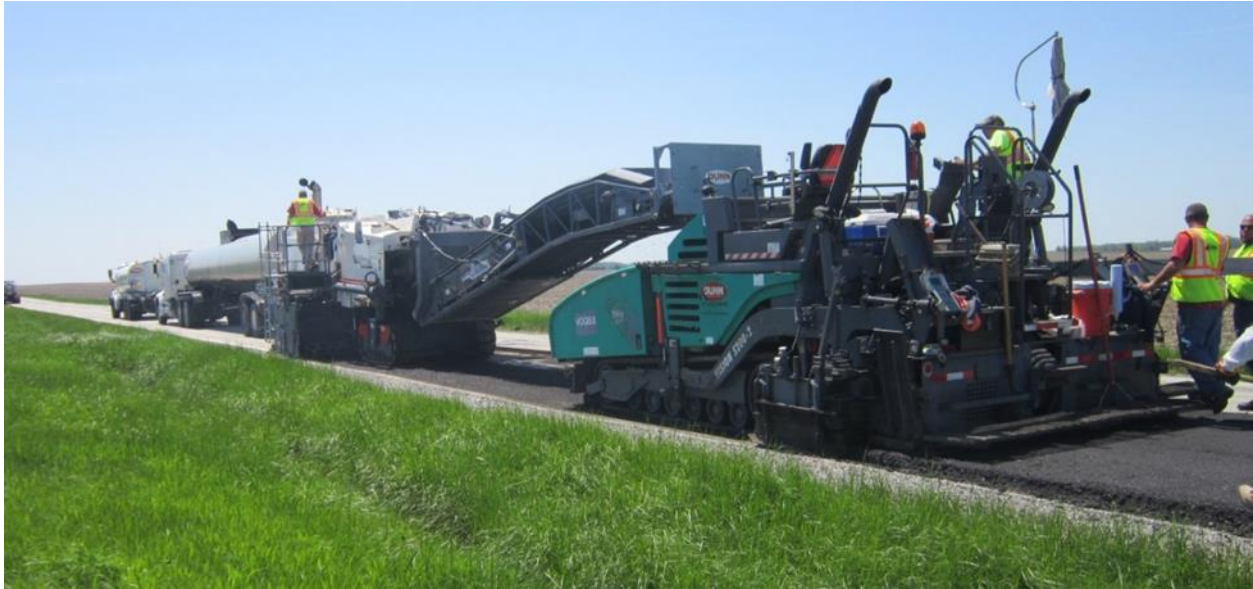
Figure 13 Single Unit CIR Train (courtesy HRG)
