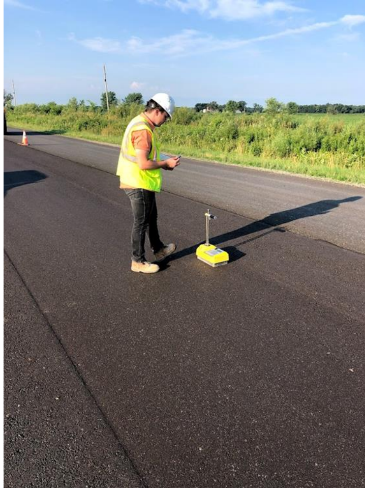
Figure 27 Nuclear Density Testing (Courtesy HRG)
